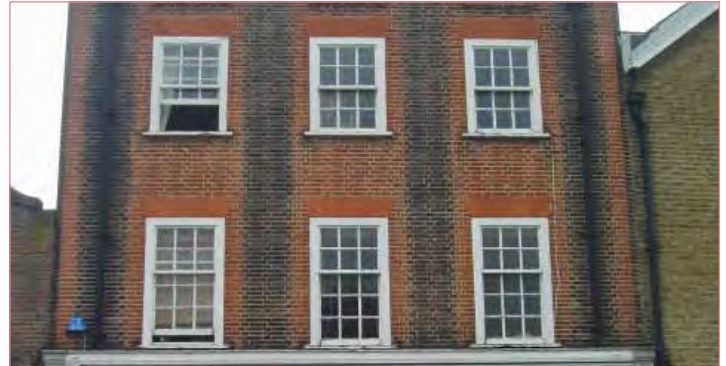
Grand 'Georgian' sash windows tend to appear on the larger scale buildings
