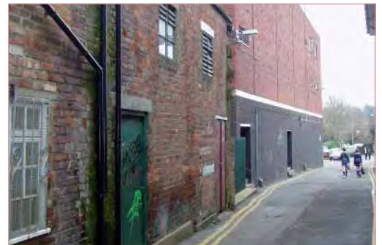
Older buildings and electricity substation next to the existing Tesco store
