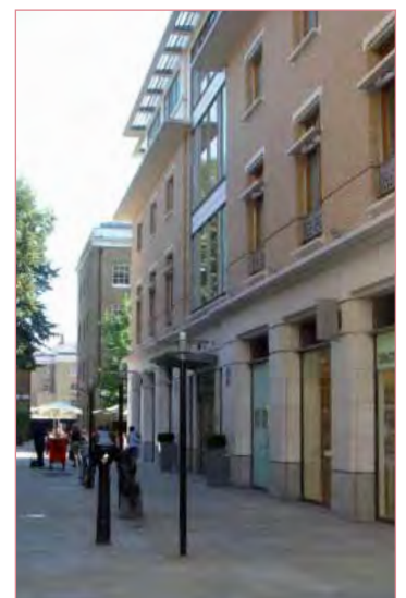
Building height should not exceed four storeys and on lanes recessed upper floors should be encouraged
