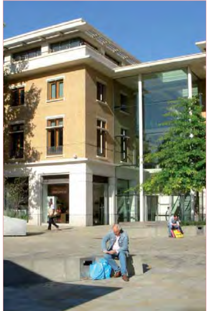
The Car Parking Square should be designed to create an attractive environment to allow the transition between cars and pedestrians
