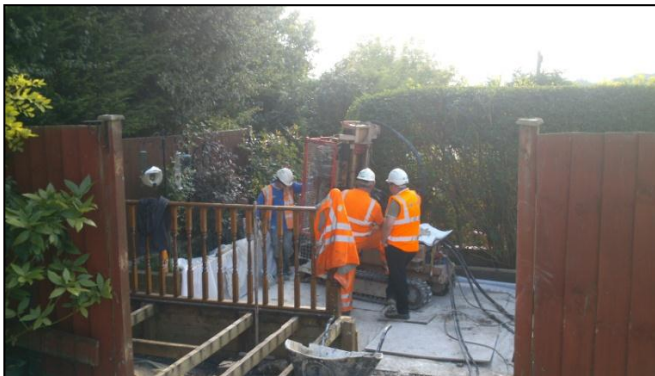
Rig Working in Meadow Rd Gardens
