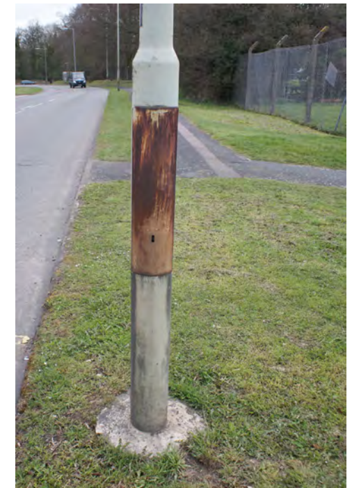
18 - Existing lighting column
